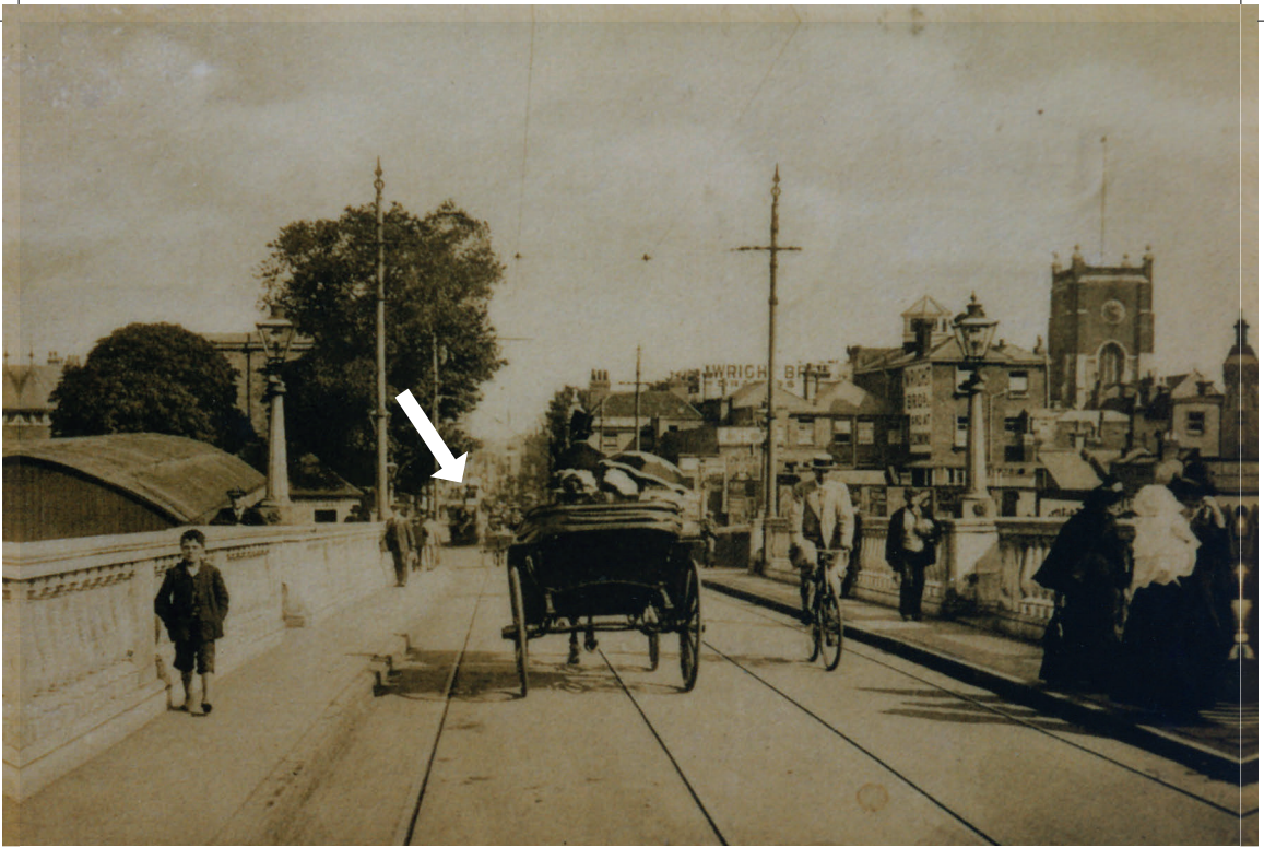
Above: The new bridge had become dangerously narrow by the early 1900s.
