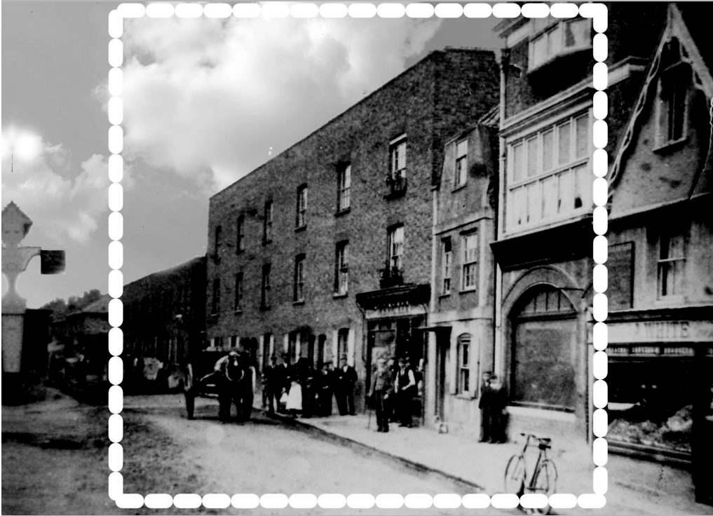
A large section of the High Street (shown dotted above) was demolished by pick-axe and sledge hammer to make it wide enough to accommodate the trams. Even before the rubble had been removed, the tramlines are in place and two men are already fixing the overhead wires whilst a gang start to lay the jarrah wood blocks imported from the Swan River near Perth, Western Australia that will finally provide a mud-free surface for the convenience of other traffic and pedestrians.
