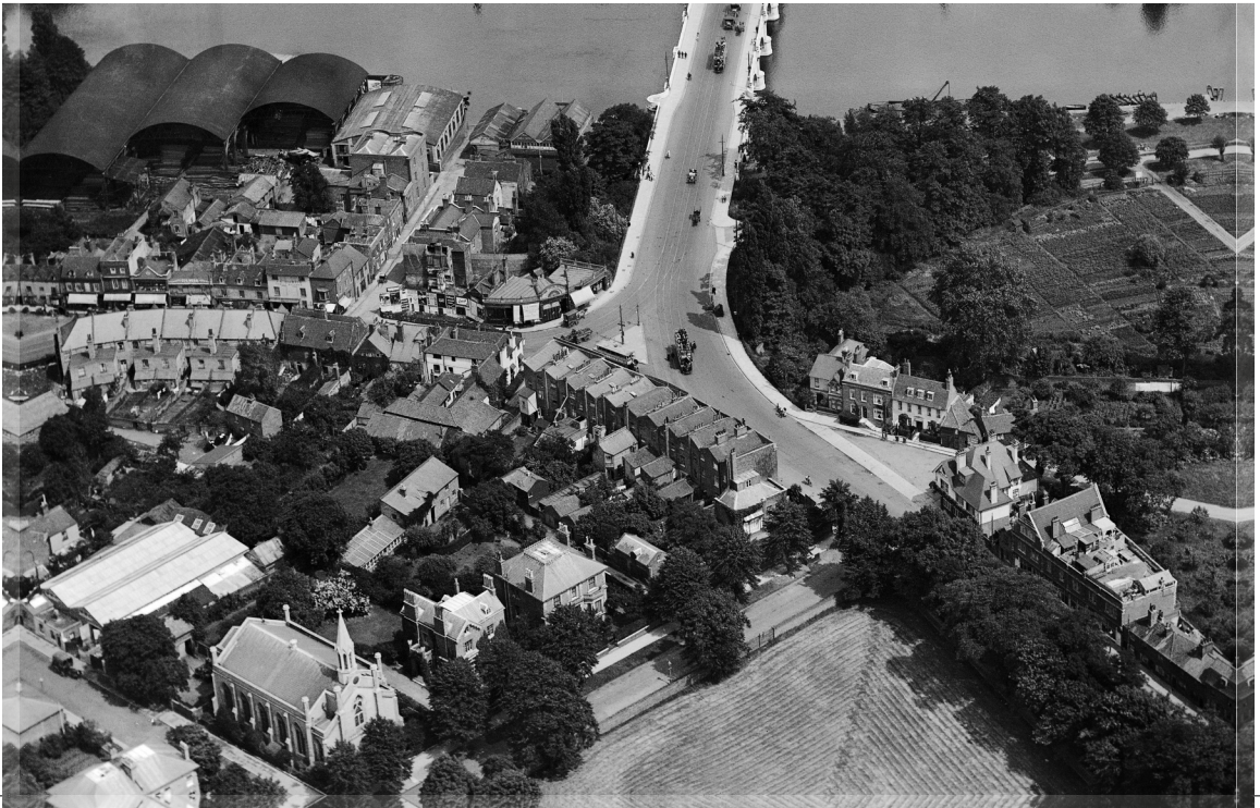
Below: An aerial photo taken in 1920 shows the extra capacity of the hugely widened bridge deck.
