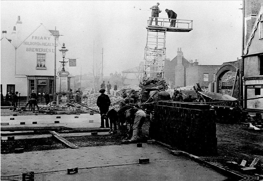
A large section of the High Street (shown dotted above) was demolished by pick-axe and sledge hammer to make it wide enough to accommodate the trams. Even before the rubble had been removed, the tramlines are in place and two men are already fixing the overhead wires whilst a gang start to lay the jarrah wood blocks imported from the Swan River near Perth, Western Australia that will finally provide a mud-free surface for the convenience of other traffic and pedestrians.
